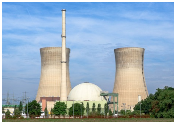
Nuclear power station - Germany
